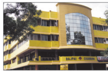
Bajpai Chambers Rajendra Nagar Chowk
